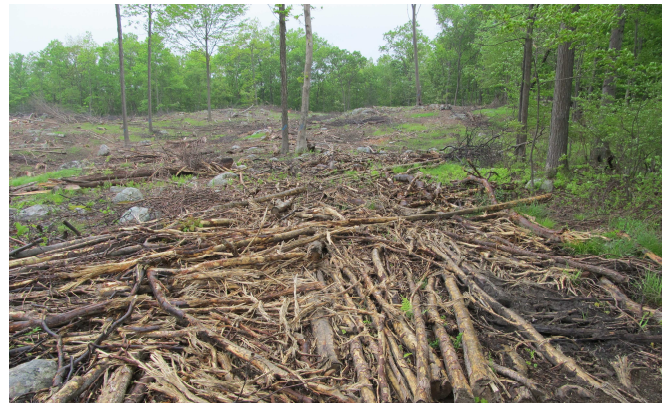
Log corduroy roads are constructed to cross wetland areas and minimize damage (Don Donnelly, NJA)
